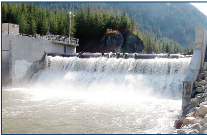
To reduce the high TDS, ultrafiltration is used in hydro power sites in British Columbia, Manitoba, and Saskatchewan potash site (see right)
