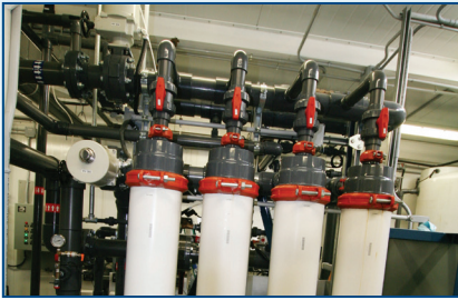
Ultrafiltration is used by a resort community on a turbid river, lowering chemical and maintenance costs
