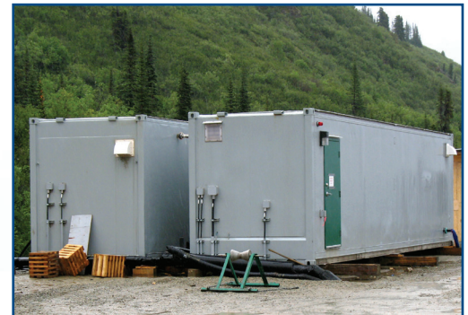
MBR sewage and water treatment package plants at Yukon Zinc
