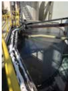
Cyanide destruction process underway in tank
