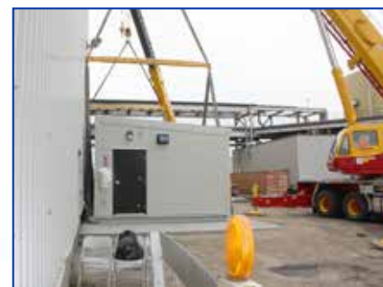
Secondary process water treatment plants for coal power utility, Transalta
