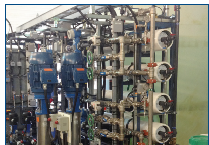
RO unit recycles wastewater at a remote oil & gas camp, saving a half million dollars a year in wastewater disposal
