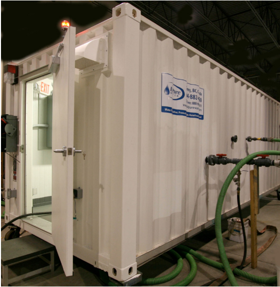
The water treatment system is housed in an easy to move, insulated shipping container.
