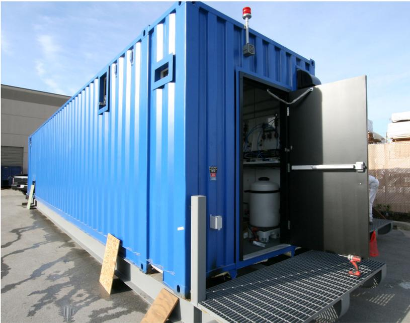
*The package water treatment buildings are new insulated shipping containers to easily transport to different sites*
