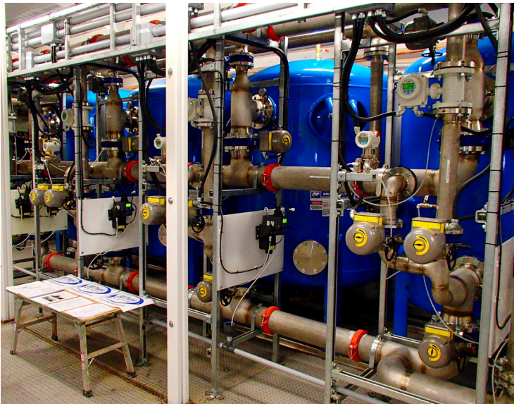
Four parallel media filters use silica sand for filtration of particles. Turbidity meters monitor the water.
