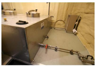
Stainless steel water tank and propane heater inside the insulated container
