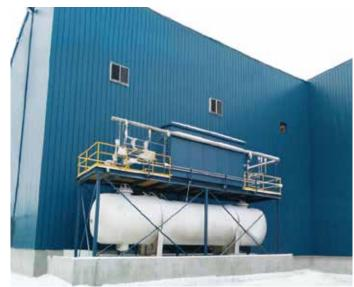
The liquid SO<sub>2</sub> control building with storage tank located at Phoenix Gold mine (above), and the portable insulated gas handling huilding built at the Process Manufacturing factory
