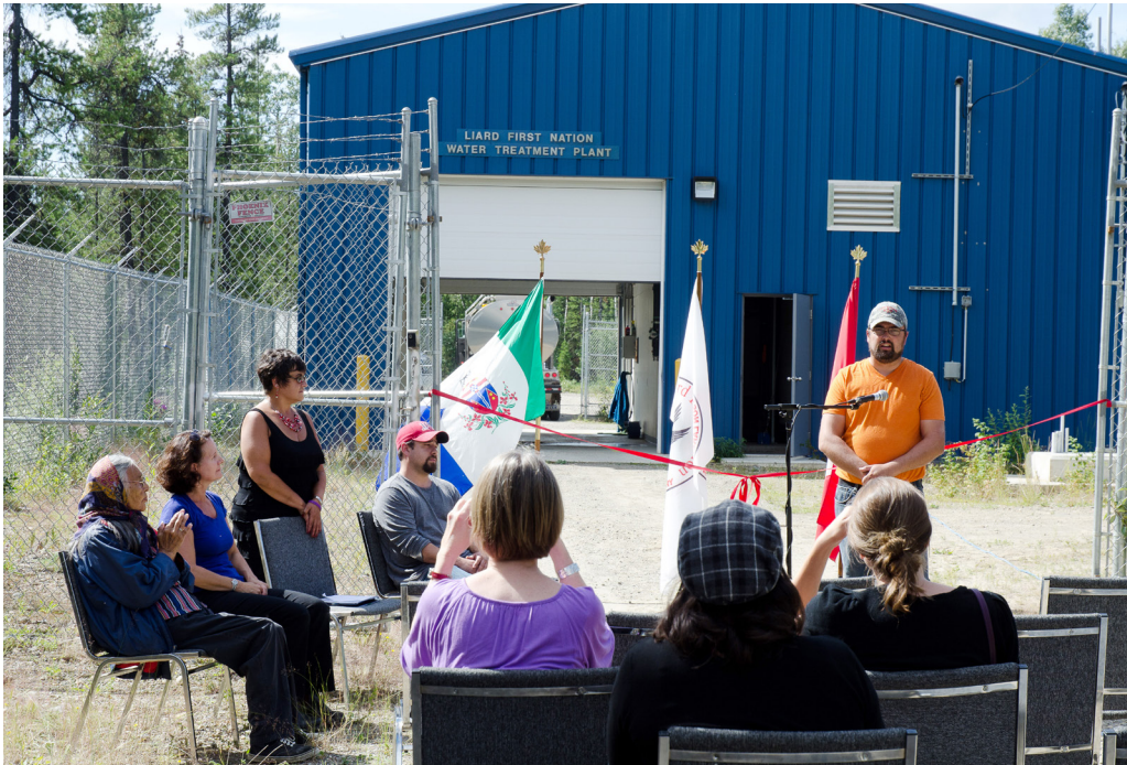
The community celebrates the new truckfill and water treatment plant
