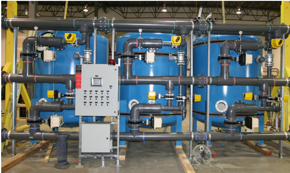
The three steel Greensand media vessels are piped in parallel at the Watson Lake treatment plant, right
