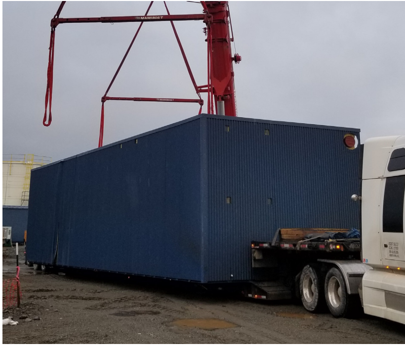
Fig. 7 – 200 cubic meter insulated and clad coated carbon steel EQ tank loaded for transport.
