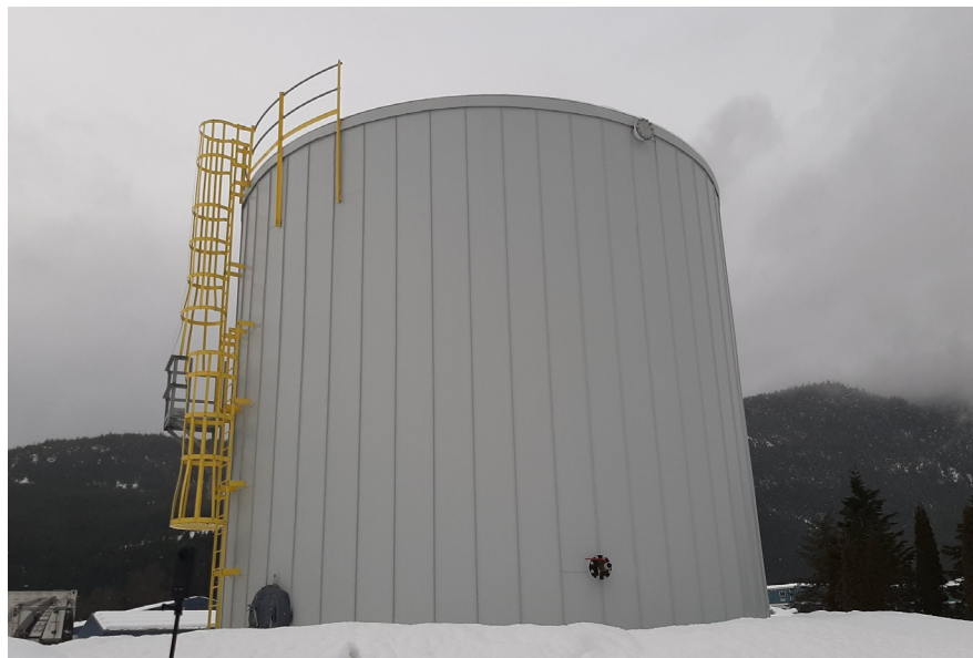
Fig. 4 - 400 cubic meter bolted, insulated and clad potable water tank for Kitimat construction camp.
