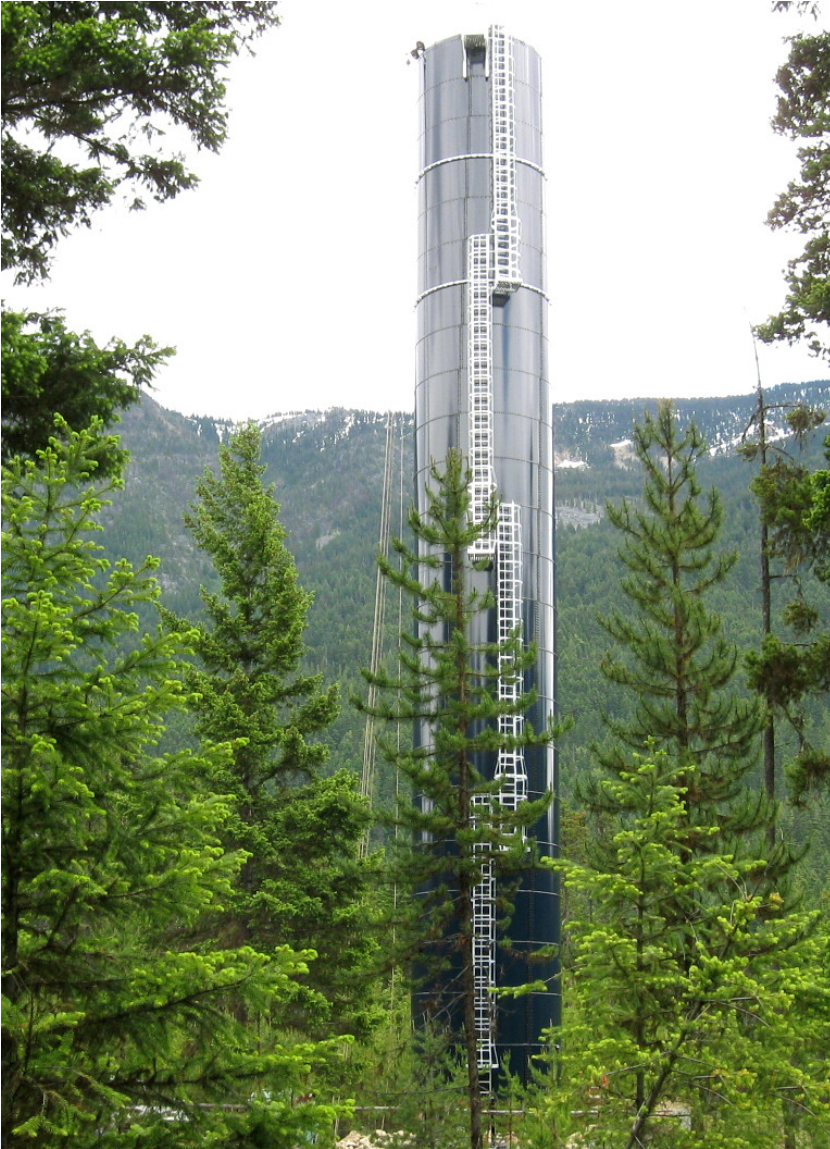
A 33.5M (110 ft) Stanco reservoir provides storage and pressure to the distribution system.
