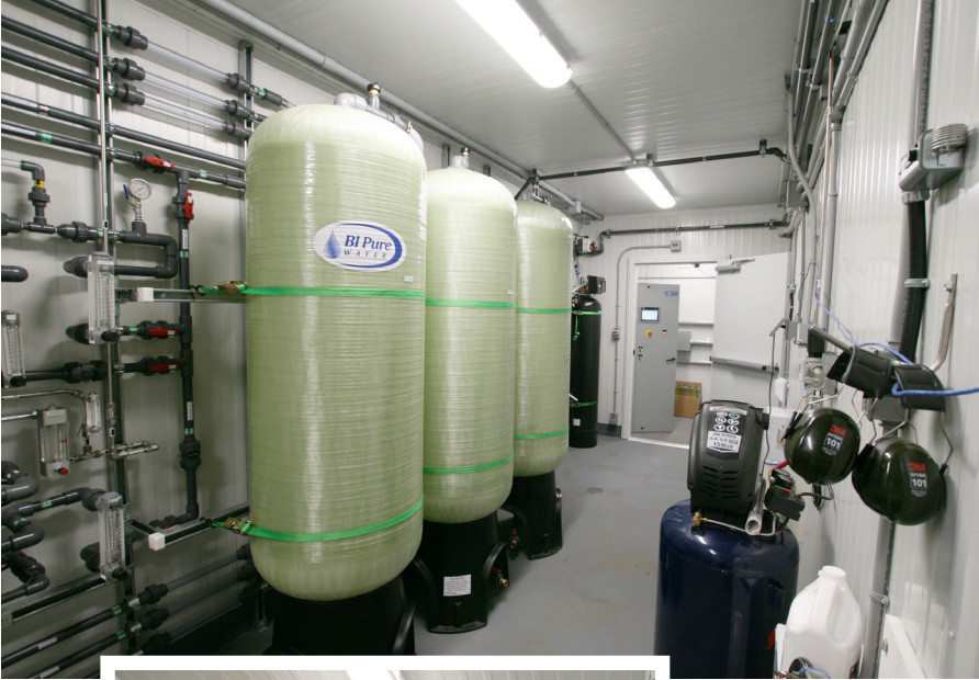
Above: Biological exchange vessels with manual flow meters and backwash piping
