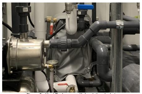
Figure 3 - Heat Exchanger with Insulation Jacket
