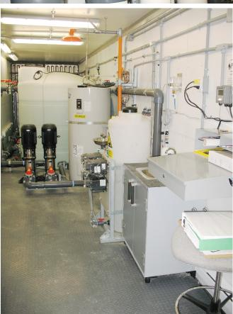
The treated water storage tank, distribution pumps, and chlorine injection system with chlorine analyzer at far right of photo
