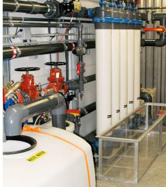
**September 2009** After two years of piloting, an ultrafiltration water treatment plant for the community of Rushmere, BC, was delivered. Located close to the Alberta border, this resort village draws surface water from Lake Windermere. The water has high turbidity levels and high amounts of organics.
