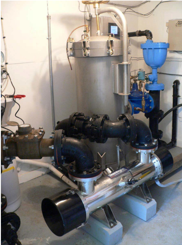
Filtration and an R-Can Municipal UV System for flows up to 1136 LPM (300 USGPM)
