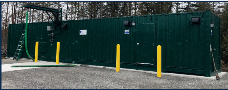
Figure 1: Exterior after installation
