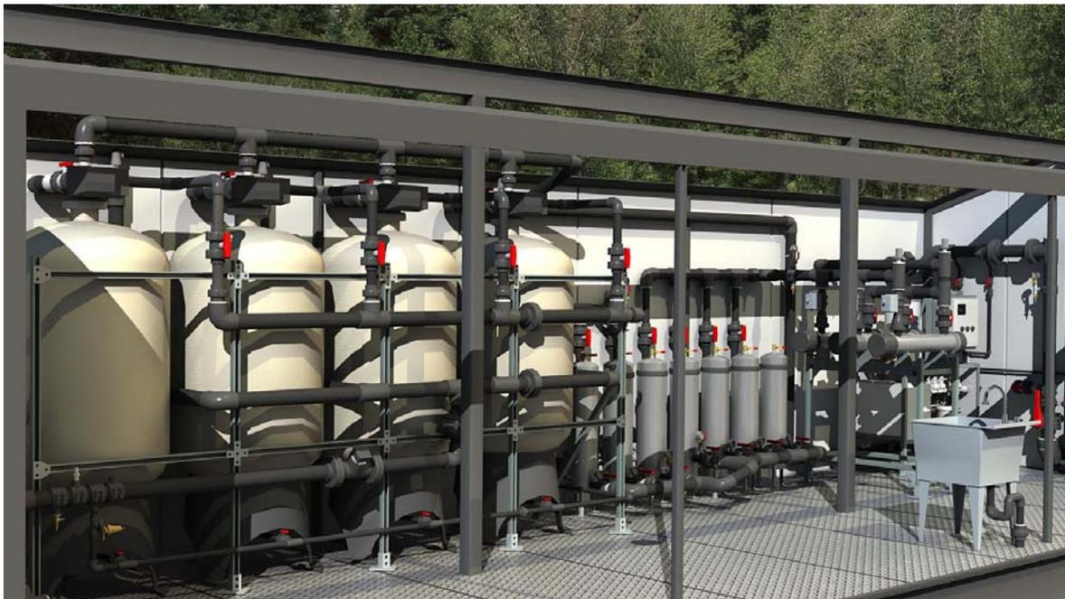
**Figure 2** - The water treatment process includes dual booster pumps, self-cleaning media filters, 5 and 1 micron A cartridge filters, ultraviolet primary disinfection and residual chlorination.
