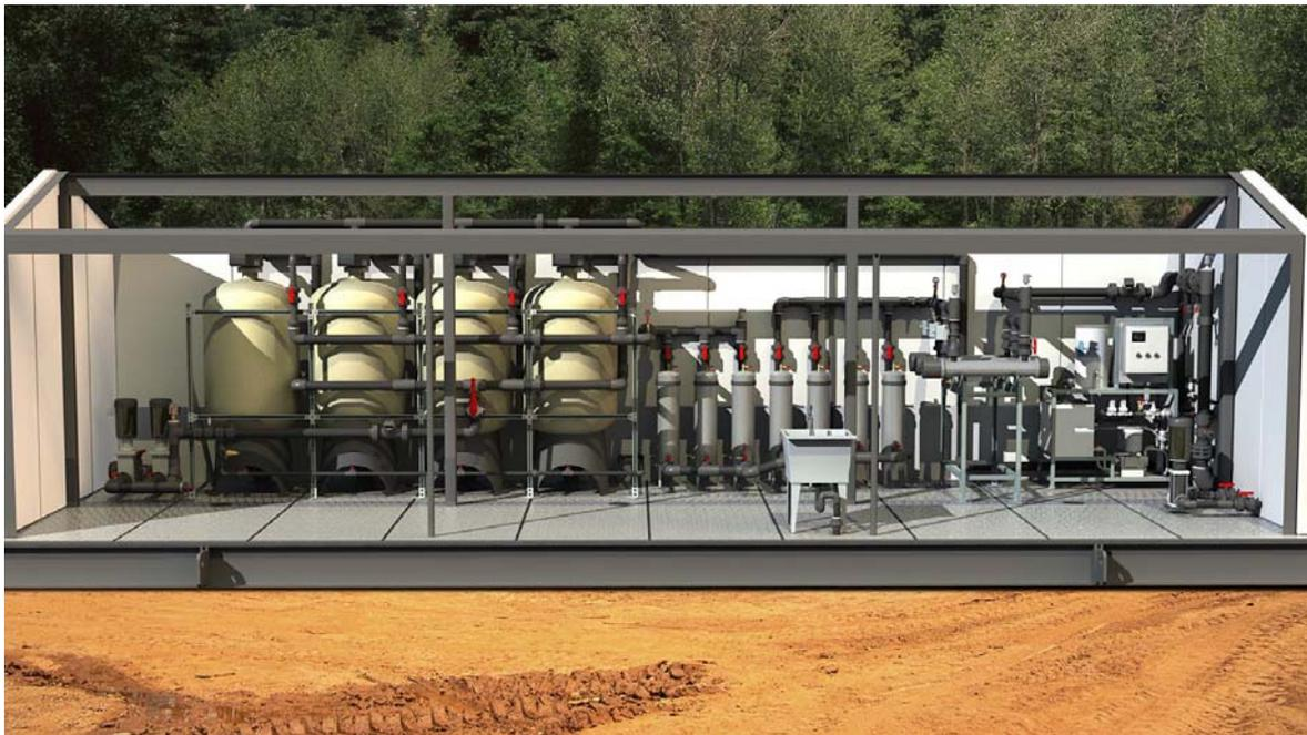
**Figure 1** - The water treatment plant was constructed on a steel skid and uses energy efficient SIP wall and roof panels.
