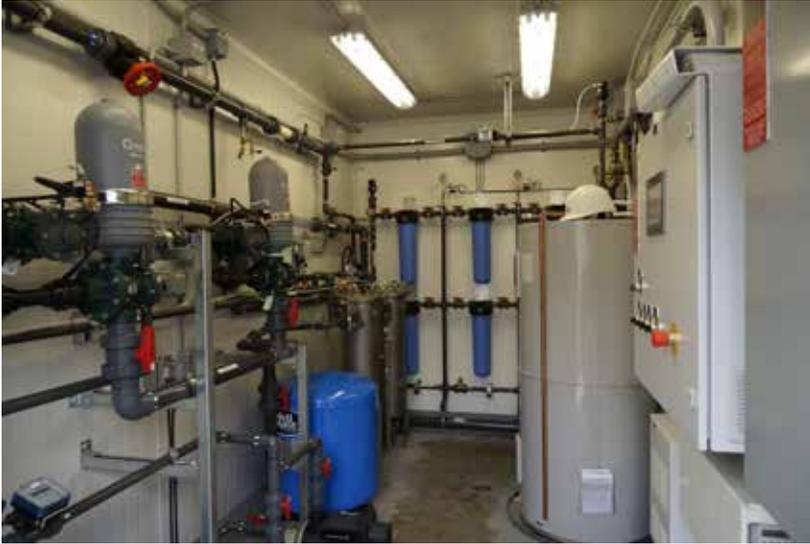
*The plant can be monitored and operated via the HMI interface on the control panel, top right.*
