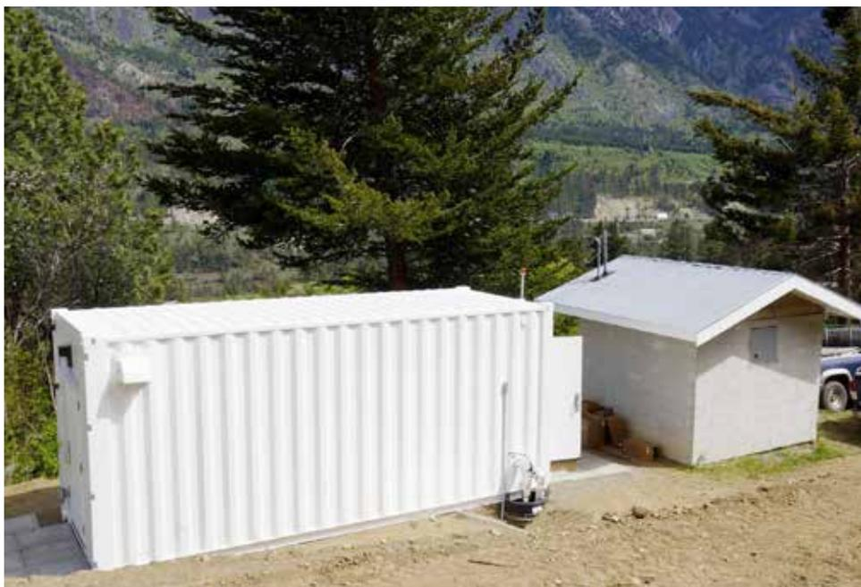
*The water treatment system housed in a modified container makes it portable and less expensive to build and commission.*
