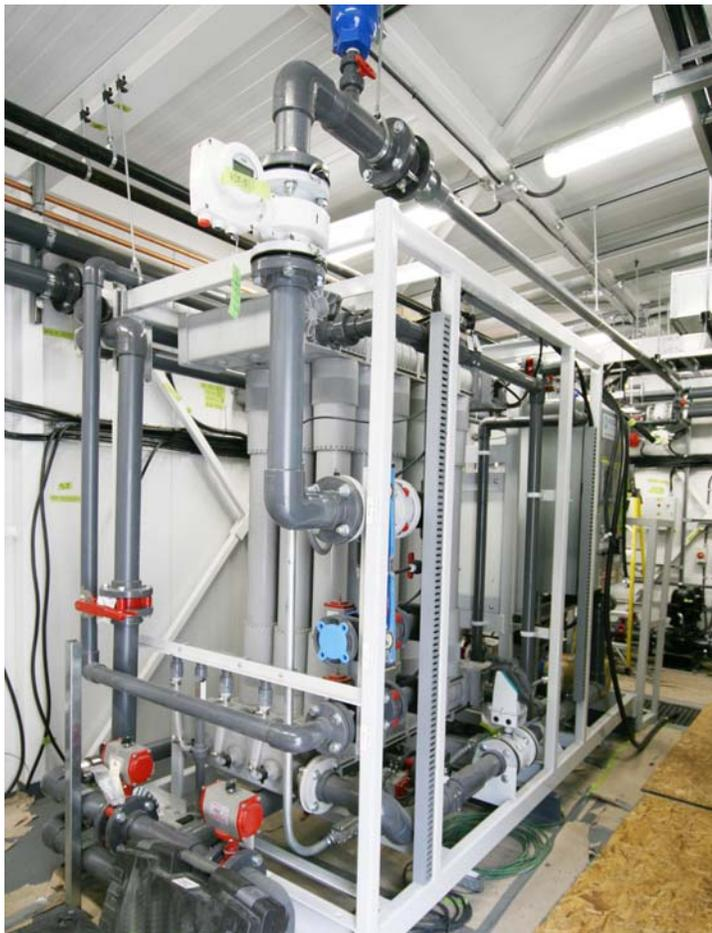
Figure 2 – The Memcor Ultrafiltration system
