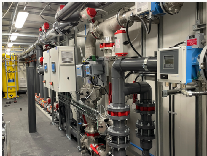
Inside of the Water Treatment Plant
