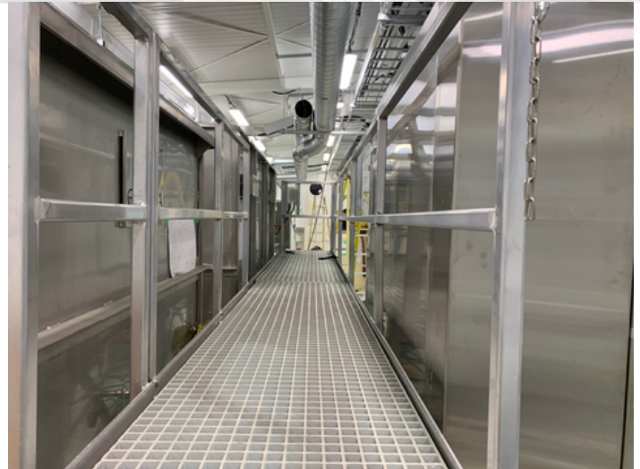
A safety walkway is installed between flocculation tanks
