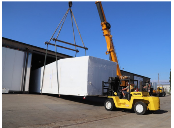
Modular Building Wrapped and Ready for Shipping
