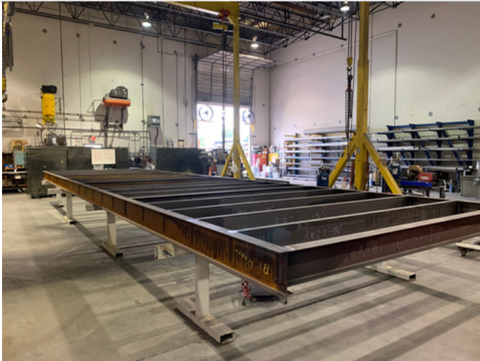
fabrication of the first steel-frame
